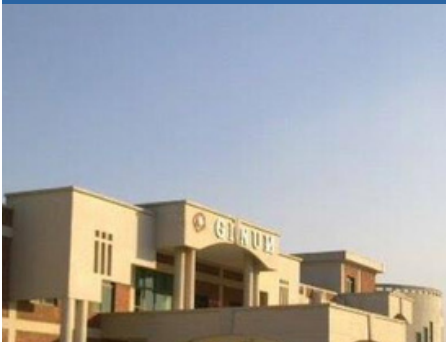
GUINUM HOSPITAL ( 500 TON )
